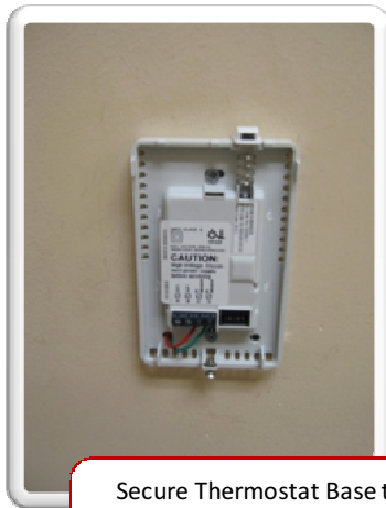
Attach Floor Temp. Sensor Cable to Connectors "C" & "D" on Thermostat Base
